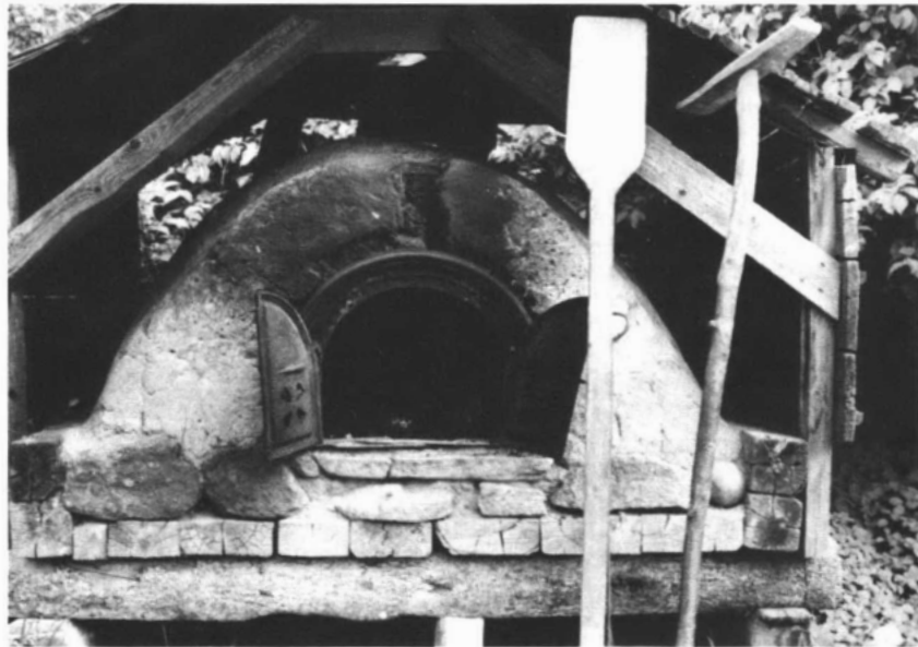
The baker's peel and the fire rake are the most used oven tools Blanchette Collection, NMC 73-25979
