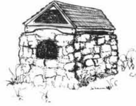
An oven with a brick dome, its sides and front protected by rough masonry Kamouraska region Blanchette Collection, CCFCS Archives, no. 194
