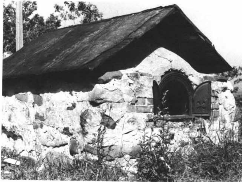
Oven with a brick dome, whose sides are protected by a wall of mortared fieldstones Kamouraska Blanchette Collection, NMC 74-14626
