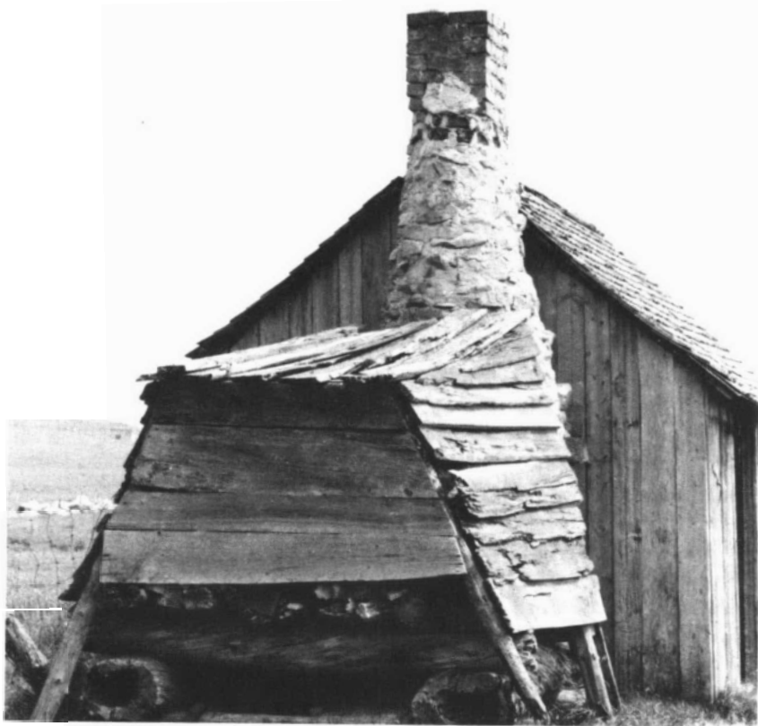
Semi-indoor oven forming part of a detached building Saint-Hilarion (Charlevoix county) Blanchette Collection, NMC 73-25993
