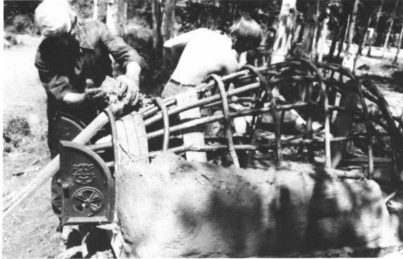
The door-frame determines the shape of the collar, or ridge Lise and Jean-François Blanchette Collection
