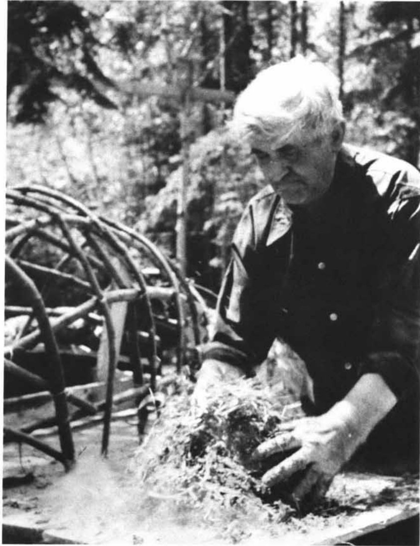
The craftsman mixes hay into the clay Lise and Jean-François Blanchette Collection
