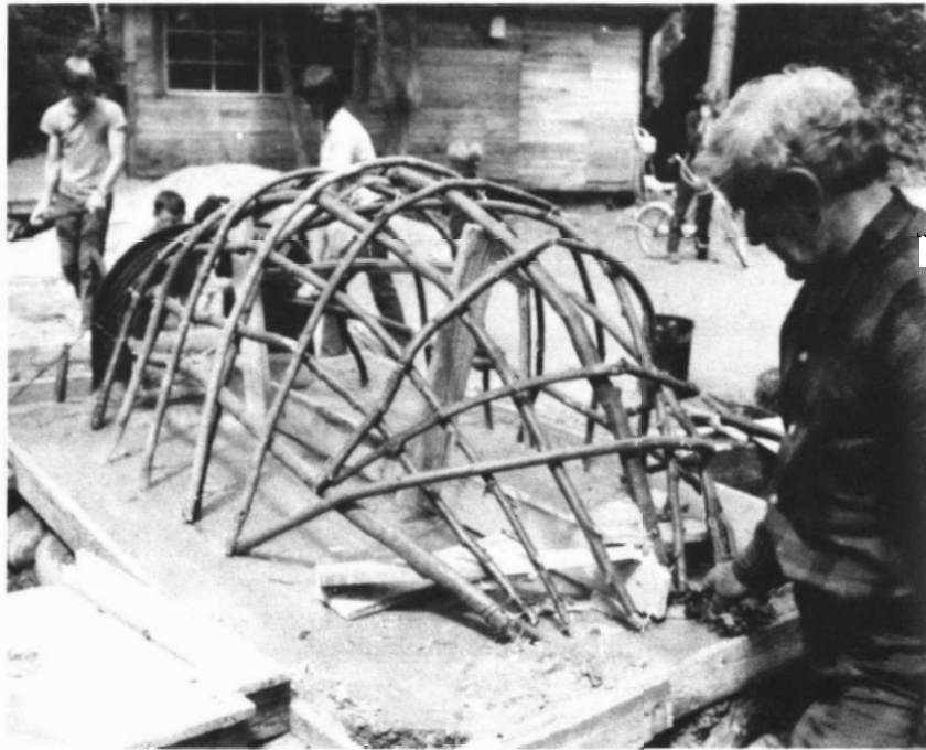
The framework reveals the eventual shape of the oven Lise and Jean-François Blanchette Collection
