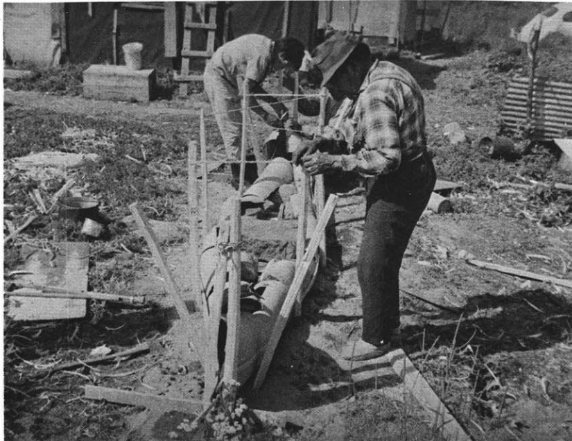
Plate 16 Tying the stakes in upright position
