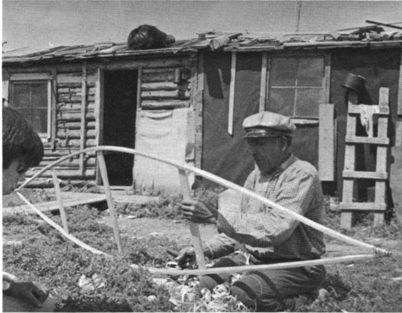
Plate 7 Assembling the gunwales and thwarts to make the building frame
