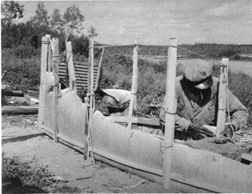
Plate 17 Internal supports and bracing laths in position
