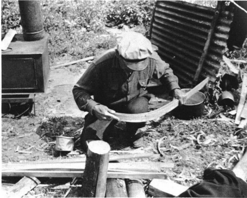
Plate 25 Bending the ribs in pairs
