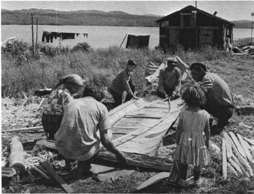
Plate 9 Centring the building frame on the bark
