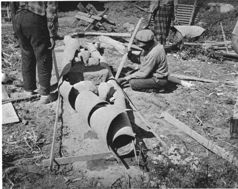
Plate 15 Placing the first stakes and lengthwise laths in position
