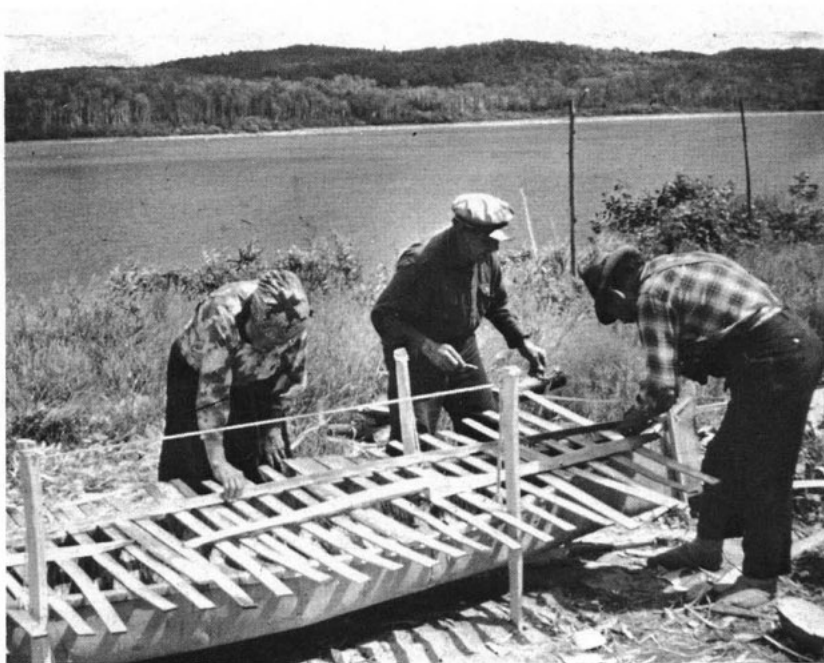
Plate 24 Marking and numbering the ribs
