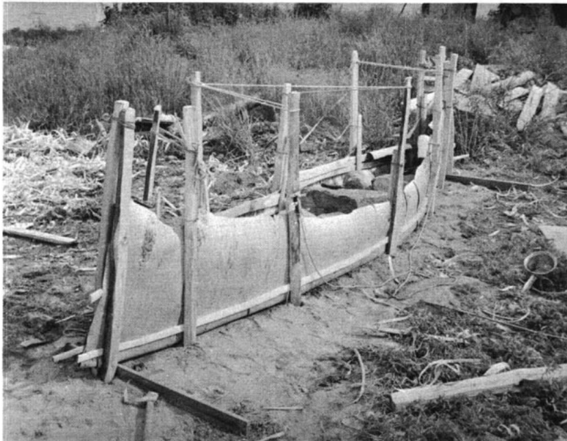
Plate 18 The complete set-up for raising and shaping the sides
