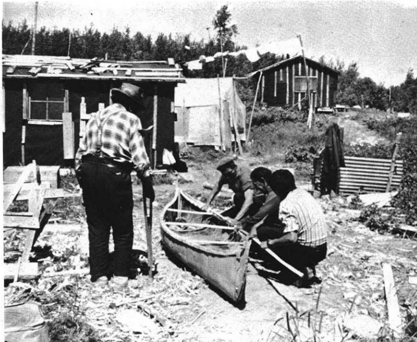
Plate 28 Installing the gunwale caps
