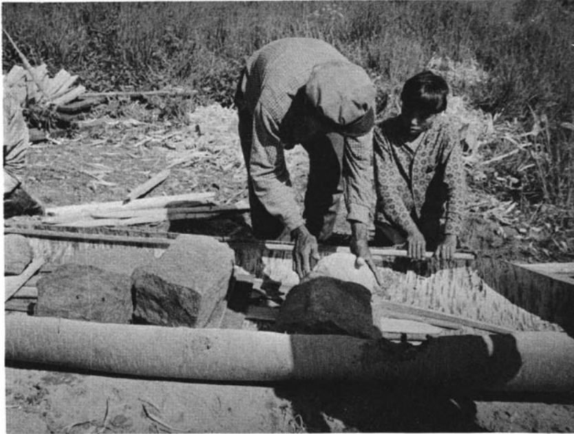
Plate 11 Weighting the building frame
