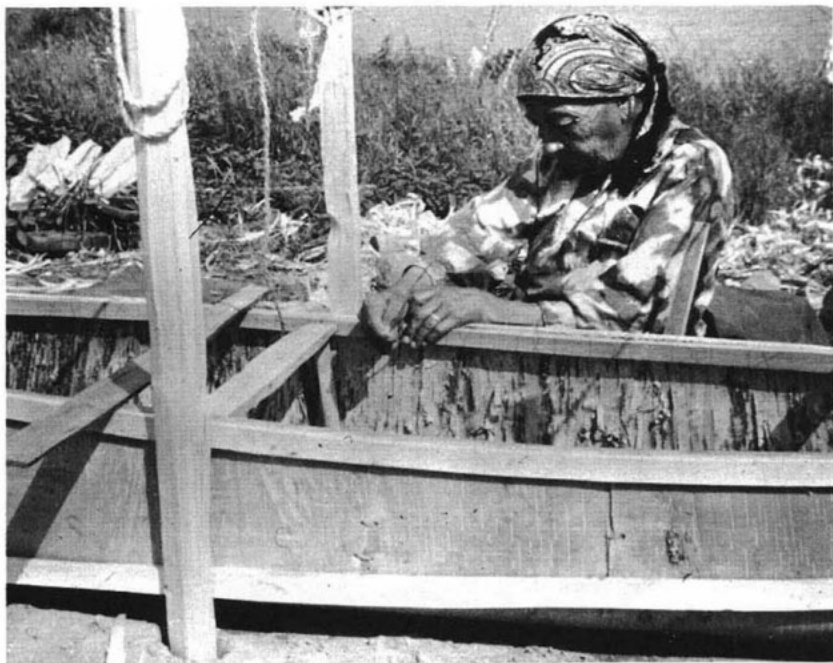
Plate 22 Beginning to lash the bark to the gunwales
